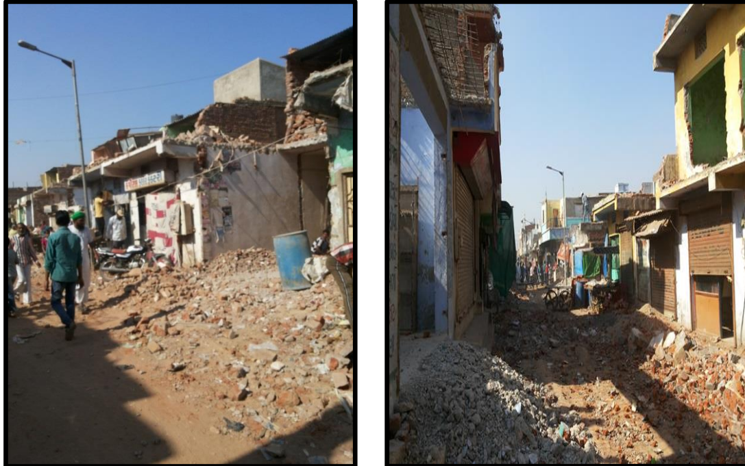
Figure 5: Demolitions on Faizal Nagar Market Road in December 2013
