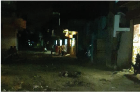
The only streetlight on this internal road is not functioning
